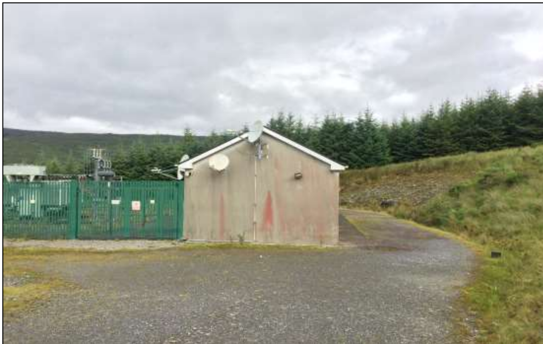
Plate 6-4 Existing substation categorised as Buildings and Artificial Surfaces (BL3)
